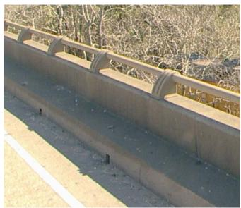
$\underline{\textbf{Combination}}$  Precast Concrete Panel on the left and Post and rail Panel on the right
